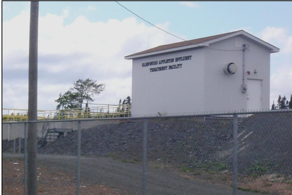
Figure 3.1 Glenwood-Appleton Wastewater Treatment Facility headworks, site of primary treatment (Photo credit: J. Daniels)
